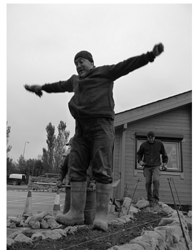
Ceri Jenkins Compacting clawdd core
